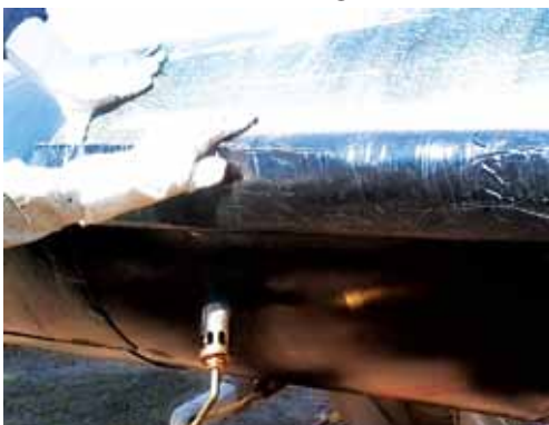
Coal Tar Tape Application
